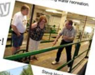
Steve Hardesty at the water treatment plant.
